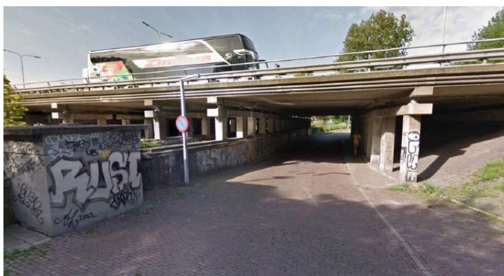
Figure 5: One of four A13 highway underpasses connecting the Delftse Hout to Delft's city centre.
