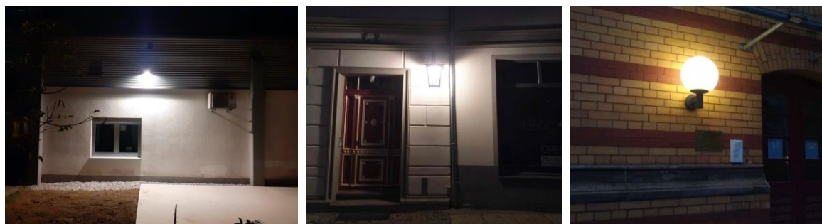
Fig. 5. Examples of photographs of “lights mounted on buildings” collected by the citizen scientists. From left to right, these are fully shielded, partly shielded, and globe style.
