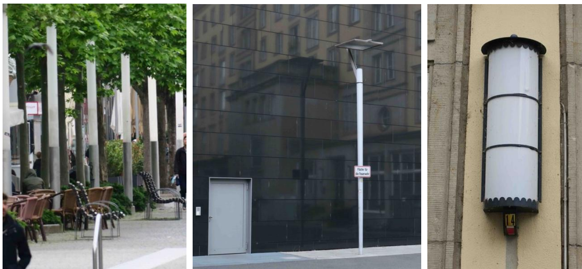
Fig. 12. Three examples of lights operated by the city of Dresden that are in the city “streetlight” database, but are not likely to be classified as streetlights by Nachtlichter participants. The light on the left should be categorized as path lighting, the light at center as either path or parking lot lighting, the light at right as a light mounted on a building. (In the case of the light at the right, the label below the luminaire clearly indicates that it is a publicly operated light.) All photos by Georg Sulzer.
