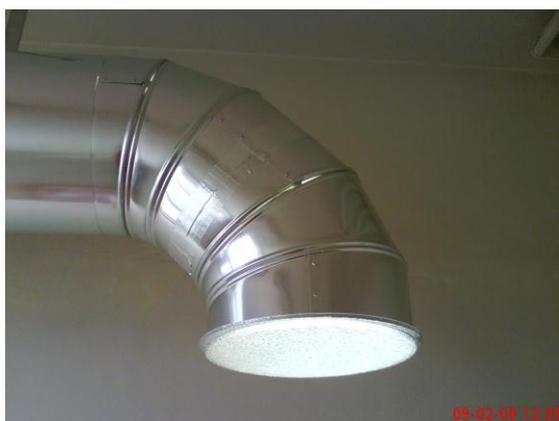
**Figure 4** Internal end of the horizontal SUNPIPE
