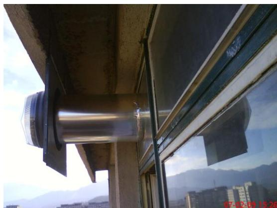
**Figure 2** Daylight dome collector of the horizontal SUNPIPE installed on the façade
