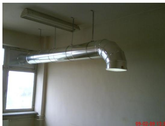
**Figure 3** Horizontal SUNPIPE ending with two 45 degrees elbows above imaginary false ceiling
