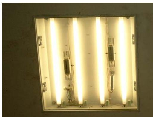
**Figure 11** Two ballasts and one capacitor are enough to operate four 18 W lamps in this luminaire very economically, both from an energy efficiency **and** from an initial investment cost viewpoint
