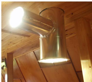
**Figure 3** Branched SunPipe prototype.
