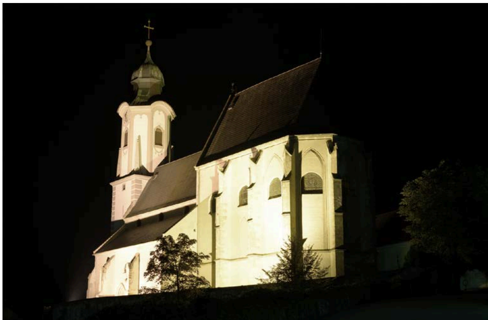
Fig. 11. Energy consumption old – 2000 watt
